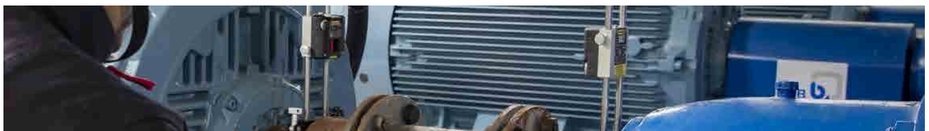
Checking shaft alignment on an electric motor with a laser system and tablet
